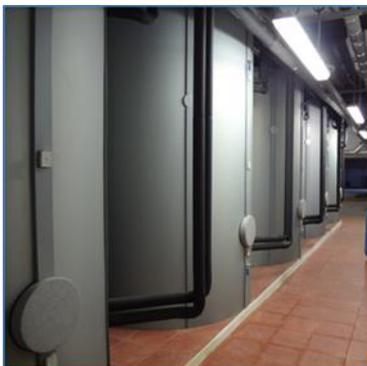
Ten new 5000-litre tanks were installed in this room, each of them with differentiated systems. Five are only inertia ones used to generate hot water for heating, and another five of inertia equipped with an internal heating coil meant for the production of hot water for sanitary use.
